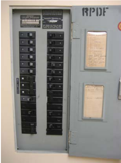
Figure 3 Location of the water chiller circuit breaker.
