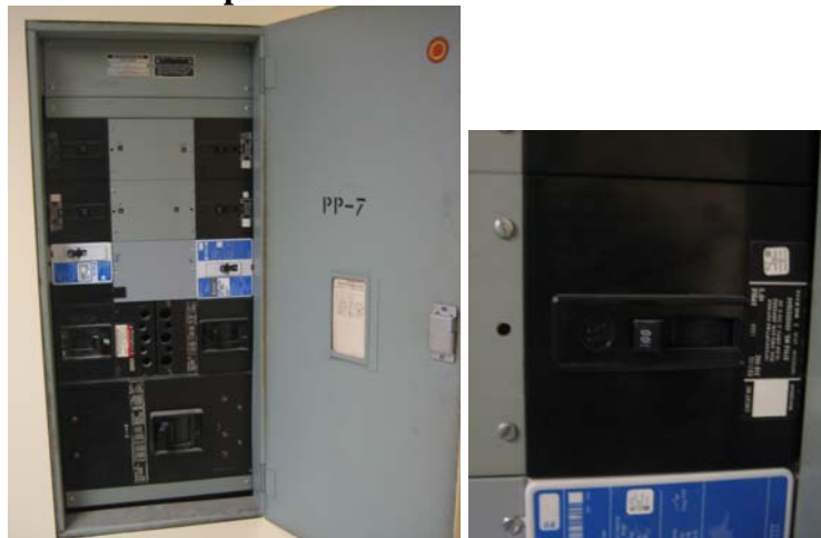
Figure 2 Circuit breaker supplying the rotating anode x-ray generator.
